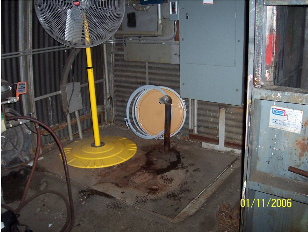
Photo 1 – Location of Pit #1 in the southeast corner of Building 51. View facing southeast.
