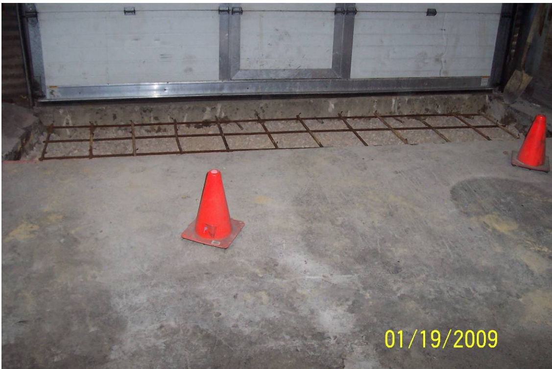
Photo 16- View of entrance slab to Building 51 with rebar. View facing south.
