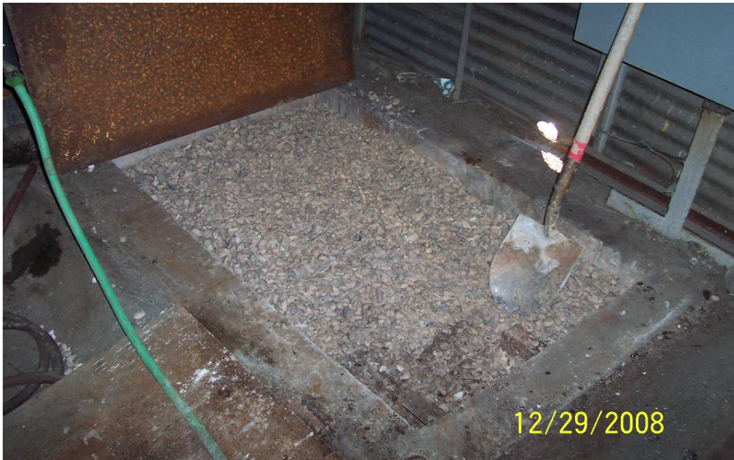
Photo 4-View of Pit#1 and sump inside Building 51 after backfilling. View facing southeast.
