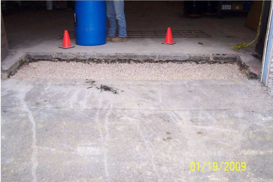
Photo 15- View of entrance slab to Building 51 after backfilling. View facing north.
